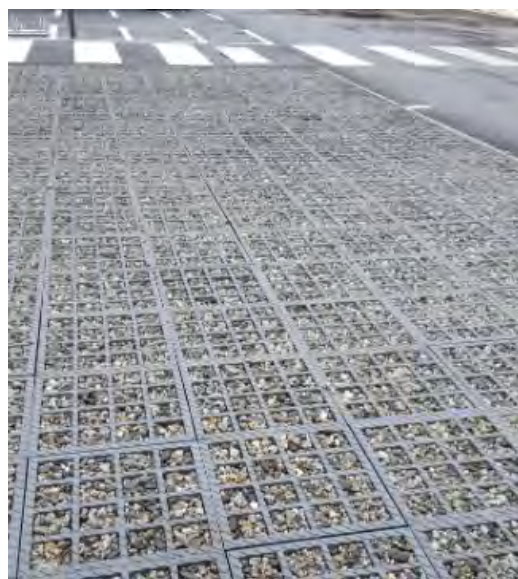
Fig. 17. Permeable surface used for a parking lot
